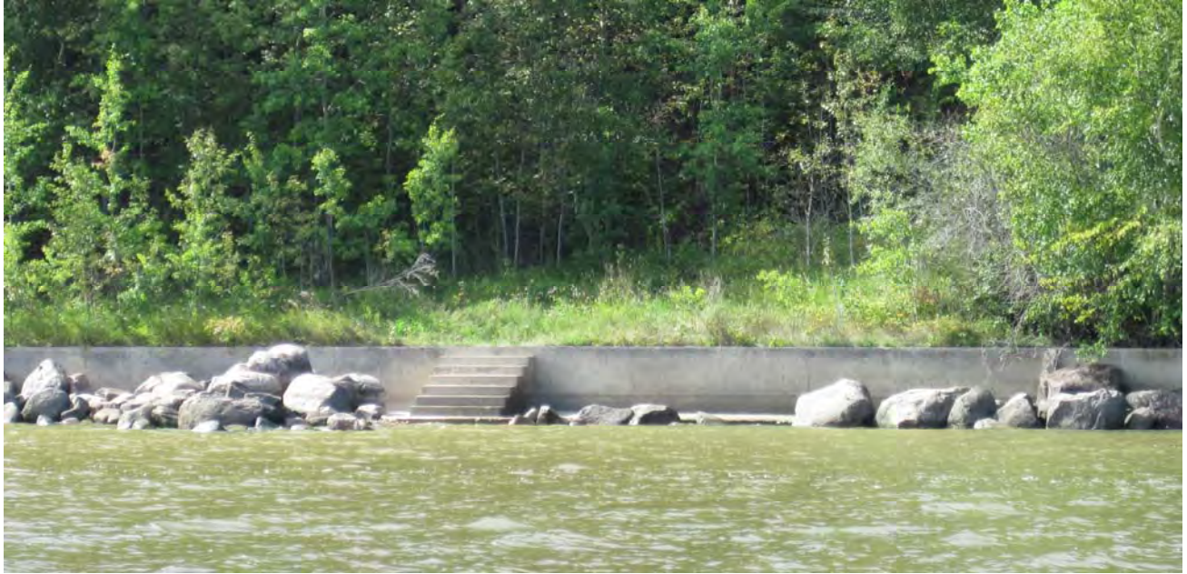
Figure 3.9 Example of Concrete Seawall
