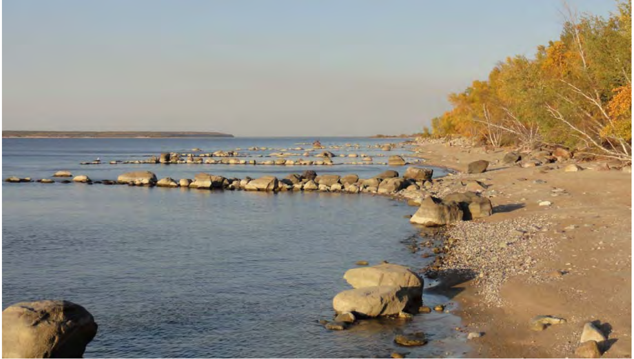
Figure 3.11 Example of Groynes (Connaught)
