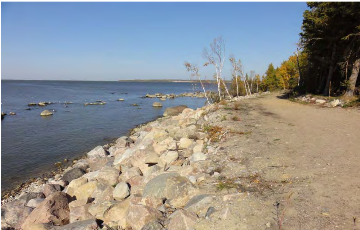
Figure 3.6 Example of Revetment (King Edward)
