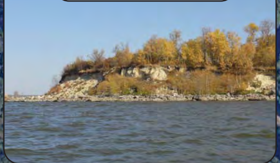
REACH 4 EXISTING CONDITIONS
