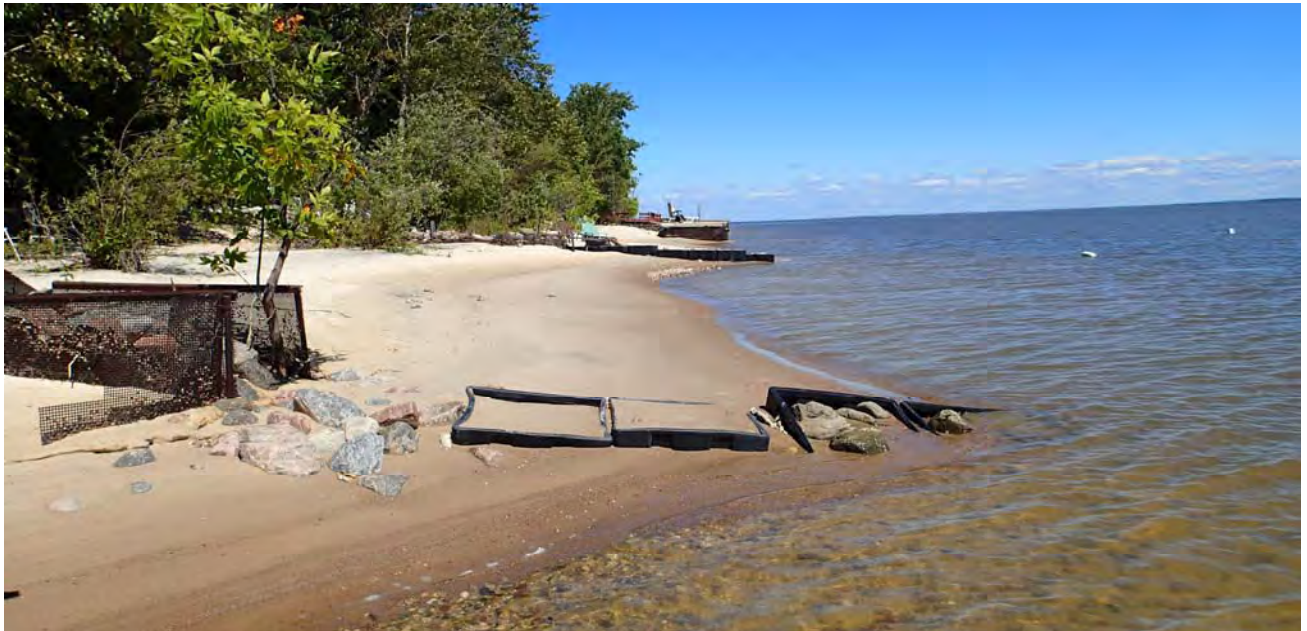
Figure 3.12 Example of Ad-Hoc Shore Perpendicular Structures along Wanasing Beach
