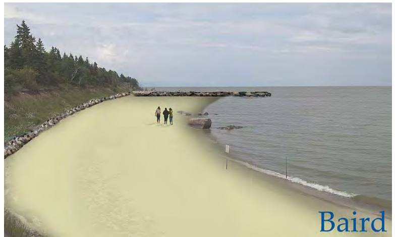
Figure 5.2 Example of Rock Groyne, Toe Protection and Slope Re-grading and Vegetation
