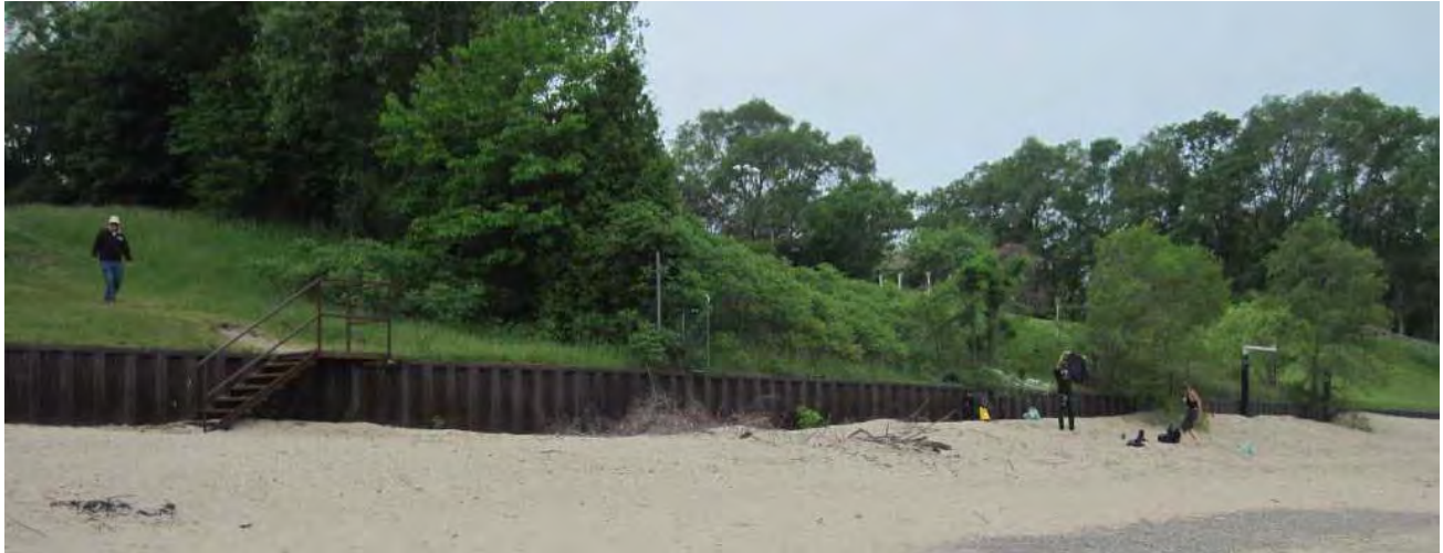
Figure 3.3 Example of Steel Sheet Pile Wall
