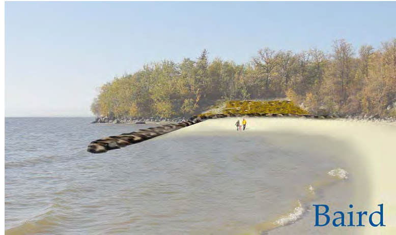
Figure 5.4 Example of Rock Groyne, Toe Protection and Slope Re-grading and Vegetation
