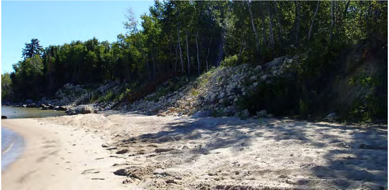
Figure 3.7 Example of Revetment (504 to Hamptons)
