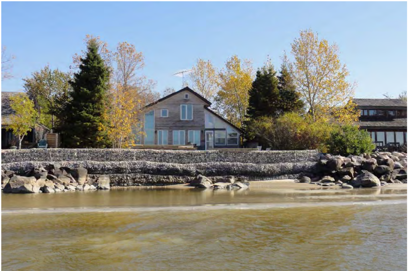
Figure 3.8 Example of Gabion Stacked Wall (Pelican)
