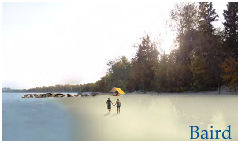
Figure 5.8 Example of Beach Nourishment with Rock Groyne
