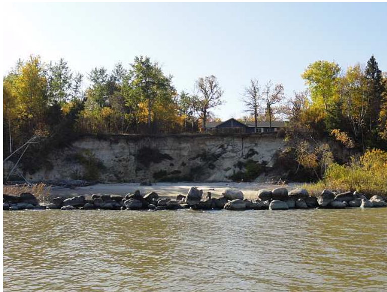
Figure 3.33 Eroding Sand Bank Where Vegetation Cleared for a Residential Lot
