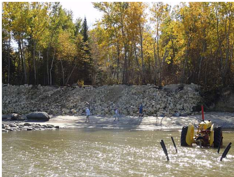
Figure 3.35 Close Up of Recent Bank Protection
