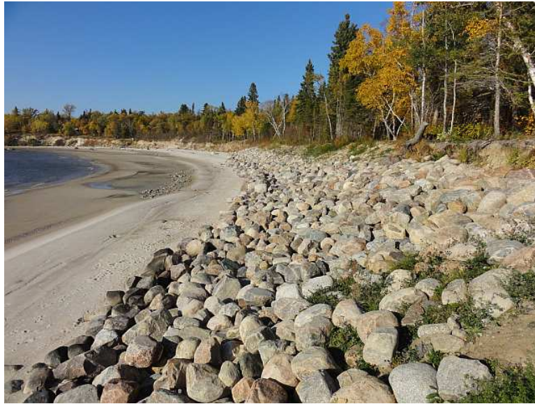
Figure 3.10 Recent Revetment Constructed at the Back of the Beach (Arthur)
