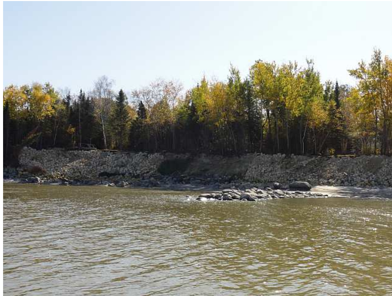
Figure 3.34 Recent Bank Protection at the Termination of Highway 504
