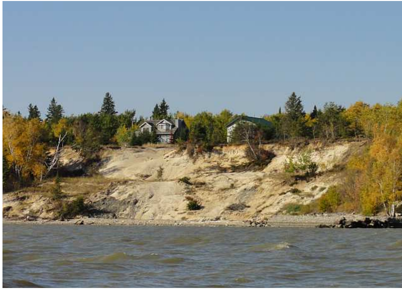
Figure 3.30 High Sand Bank with (potential) Rotational Failure
