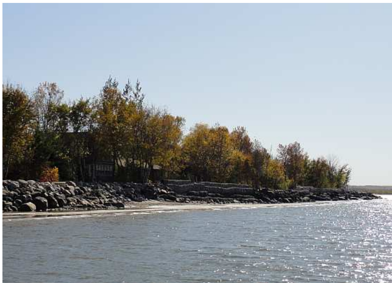
Figure 3.19 Rock and Gabion Protection at Pelican Point
