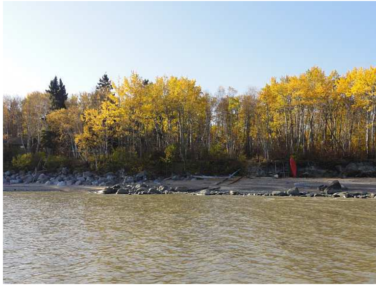
Figure 3.22 Transition from Armoured Saffie Road to Unprotected Albert Beach
