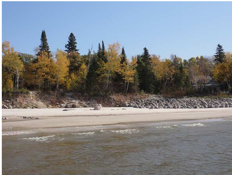
Figure 3.11 Transition from Natural Eroding Bank to Recent Revetment Shore Protection
