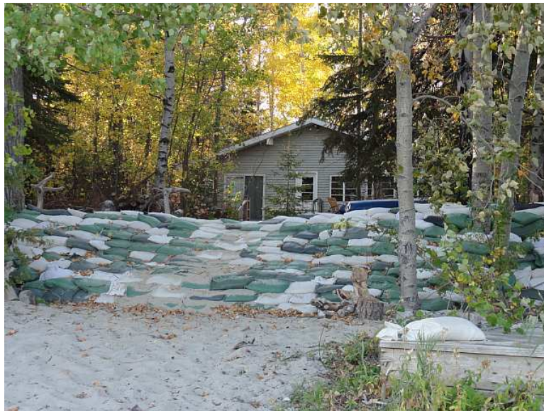
Figure 3.27 Sand Bag Dyke Protecting Flood Susceptible Homes
