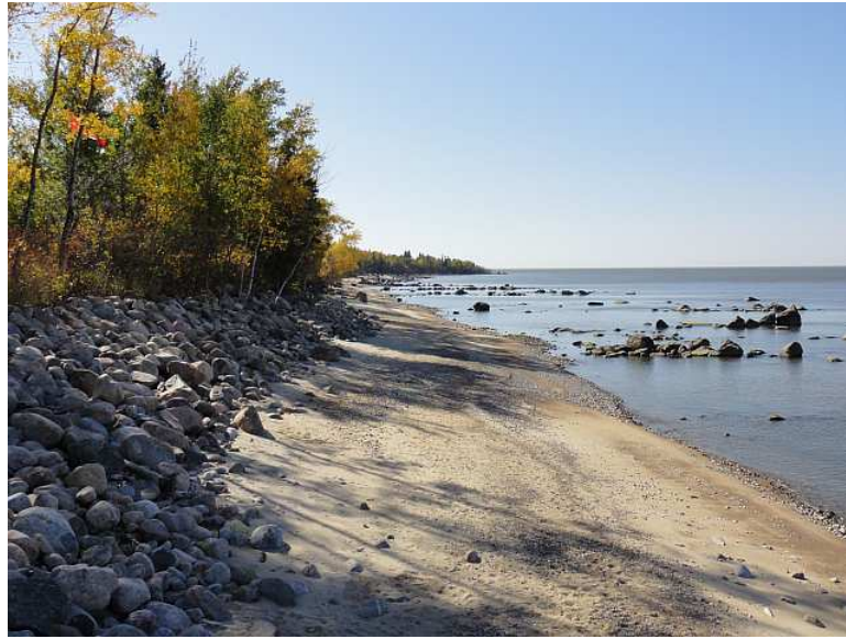
Figure 3.2 North Section of Connaught Beach Protected with a Revetment
