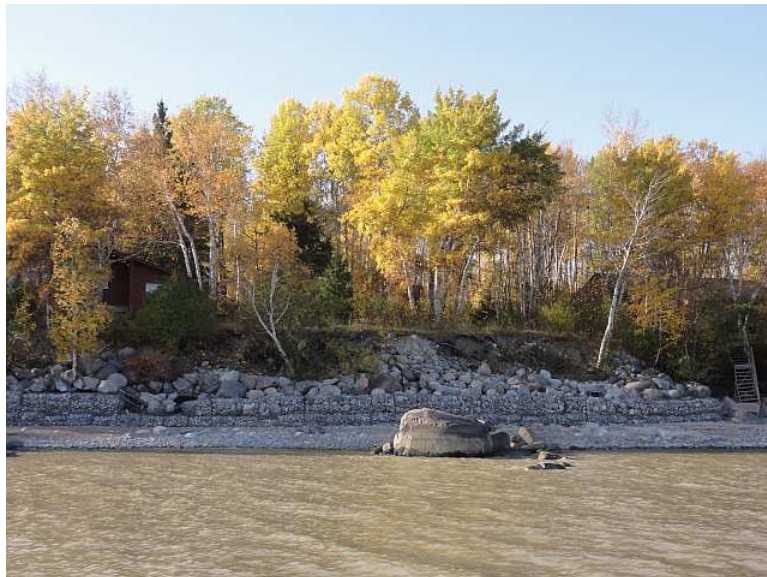
Figure 3.21 Dumped Boulders and Gabion Basket Protection
