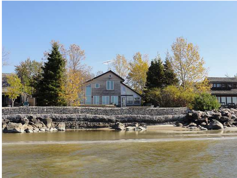
Figure 3.18 Gabion Basket Shore Protection at Pelican Point
