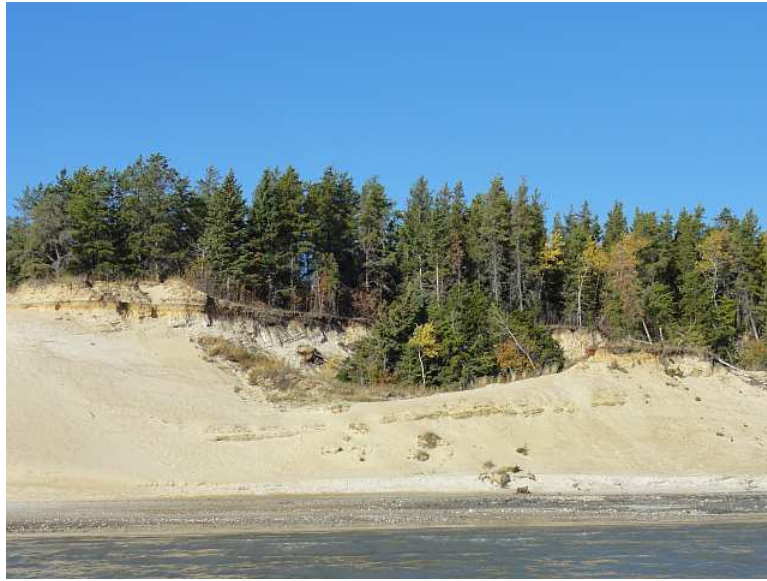
Figure 3.28 Large Rotational Failure in Sand Bluff
