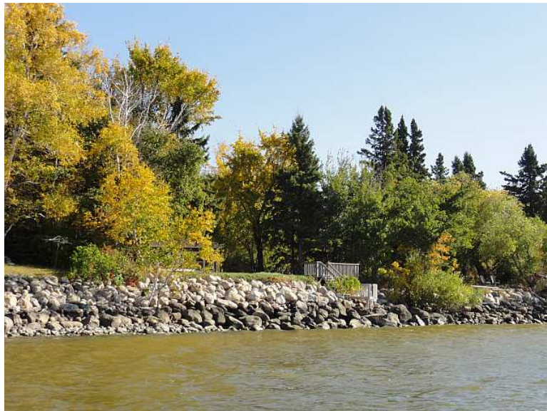
Figure 3.17 Shore Protection Along Thornton Beach
