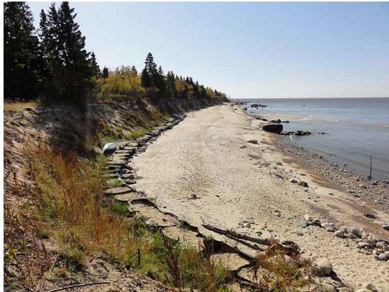
Figure 3.5 Geo-textile Sand Bags Placed at the Toe of the Bank
